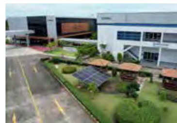
Training Village in side the plant
