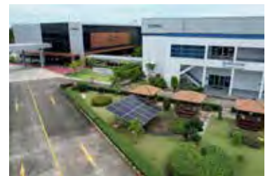
Training Village in side the plant
