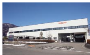
New office block at Komagane Plant (Disk Drive Suspension Div.)
