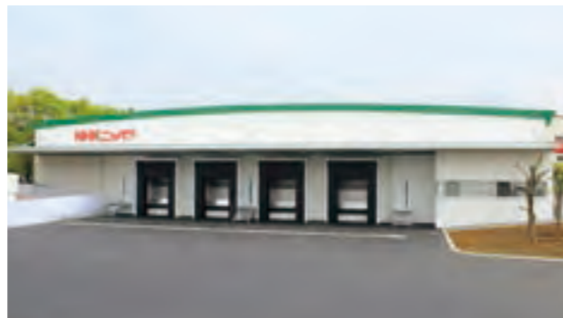
New Coverings Building at Gunma Plant
