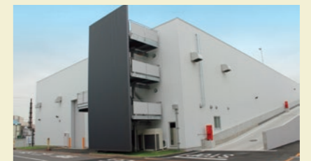
New Bldg No. 1 at the Atsugi Plant produces precision stamped products
