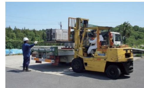
Donation of idle equipment and tools to the earthquake affected area
