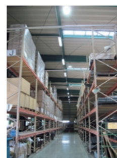
New LED high ceiling fixtures installed at NHK Sales Saitama Depot
