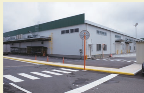
Newly finished urethane building
