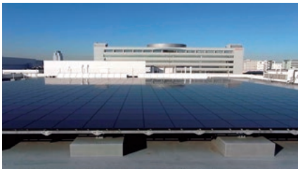
Yokohama Office (100 kW) Commissioned 2009
