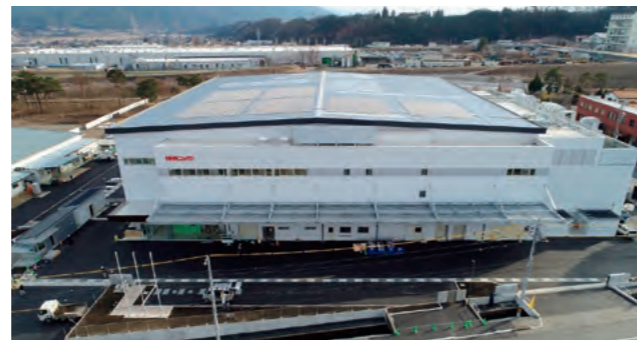
Miyada Plant (144kW, FY2018 operation start)
