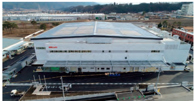
Miyada Plant (144kW, FY2018 operation start)
