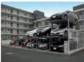
13 Mechanical multilevel parking systems These parking systems are useful in securing parking space while helping ensure efficient land use.
