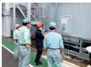
Energy saving diagnostics
