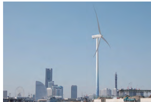
Yokohama Wind Power Plant (Hama Wing)
