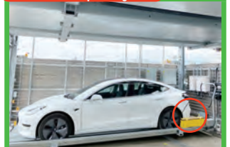
Multi-level parking lot with EV charger
