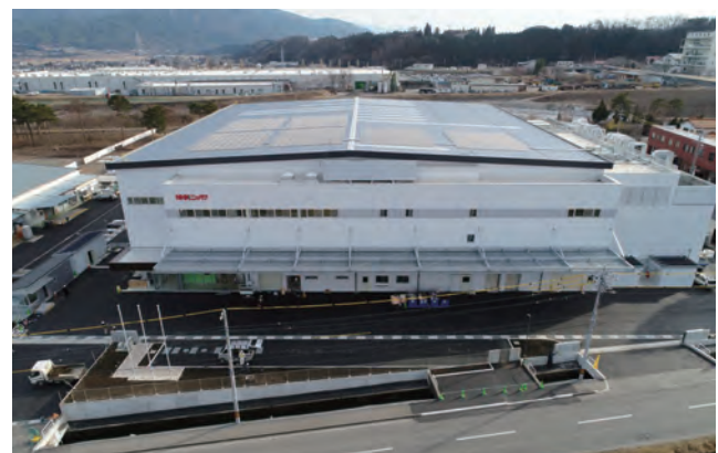
NHK Spring Miyada Plant (144kW) Started operation in FY2018
